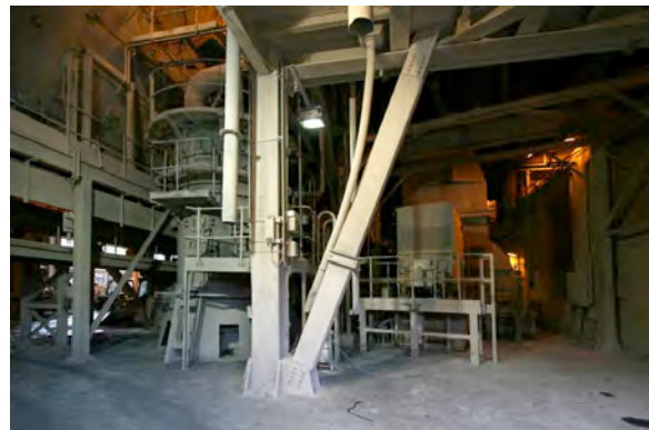
Raw material milling
